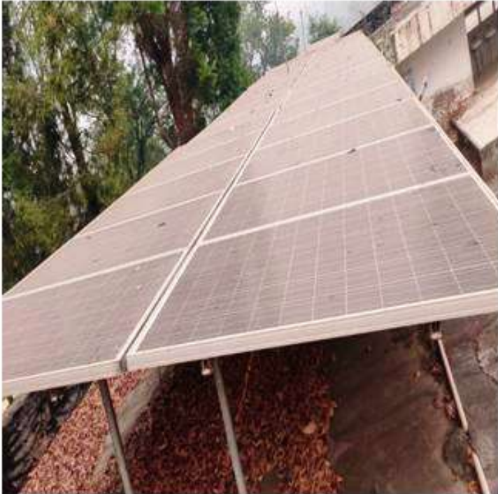
Solar Panel installed at Ladies Hostel roof
