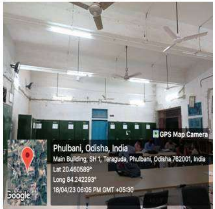
Energy Efficient LED bulbs at Library
